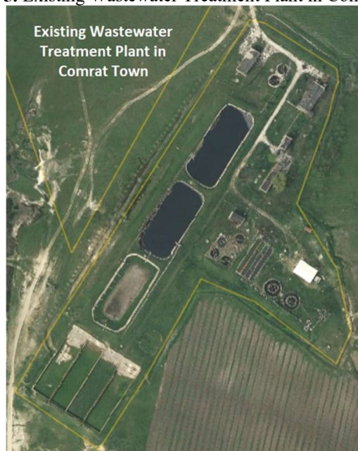
Figure 5. Existing Wastewater Treatment Plant in Comrat town
