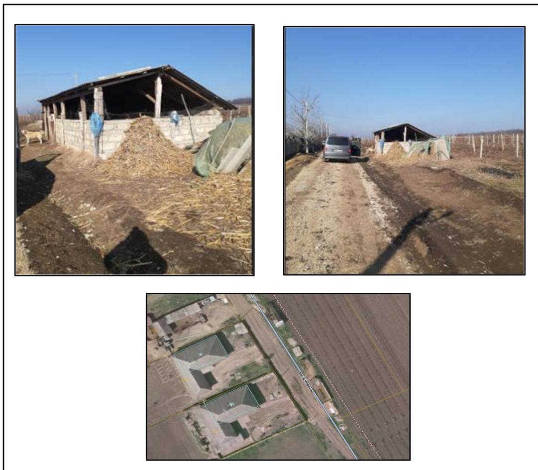
Figure 2. Warehouse located on Campilor str, in Pelinei village (17362040163) subject of possible demolition as it impedes future access to the network distribution pipes
